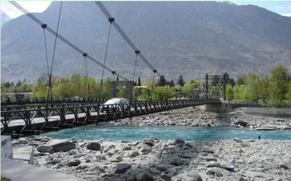
Construction of Suspension Bridge at Sakarkoi to Basin
