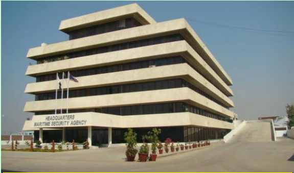
HQ MSA Building
