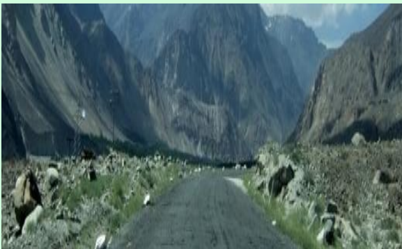
Construction of 9 km of road 16.5 feet Wide in Hunza
