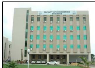
Electrical Engg. Laboratory Block at Bahria University, Karachi Campus
